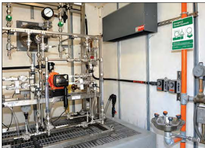
Chemical metering pumps precisely regulate the amount of methanol infused into the denitrification system.
