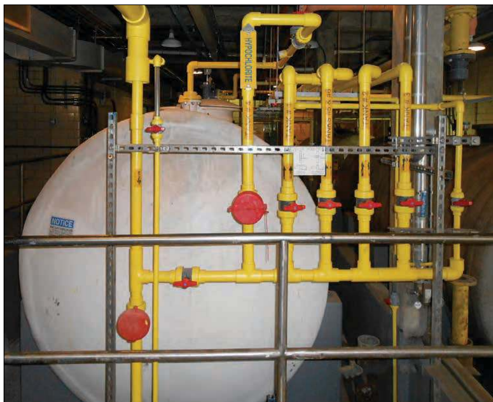
One of the upgrades to the Tallman Island Wastewater Treatment Plant in College Point is a new sodium hypochlorite tank and delivery system.
