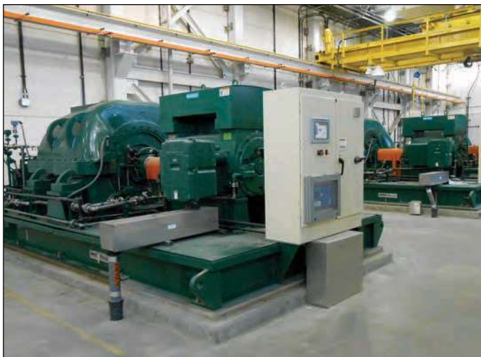
Four new blowers were installed in the air process system of the Tallman Island Wastewater Treatment Plant in College Point.
