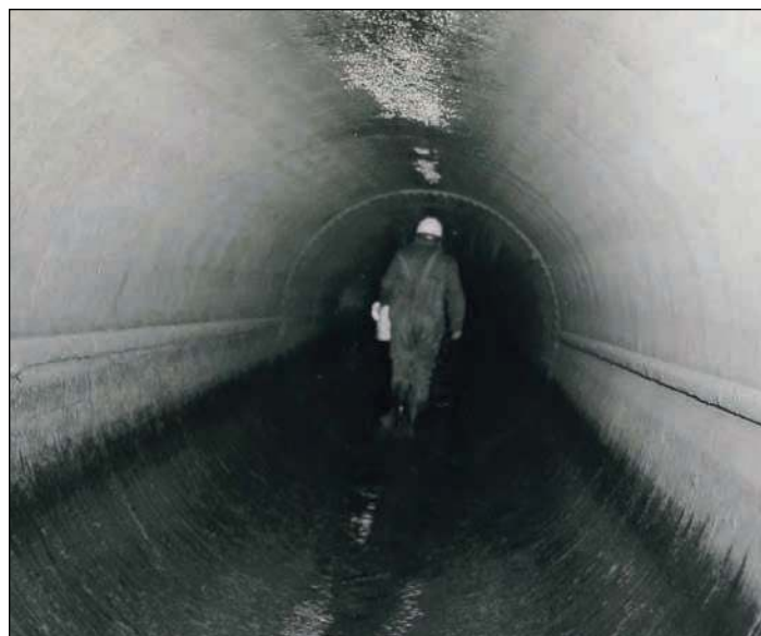
Figure 3. An inspector walks through the pipe in Seaford, Manhole No. 19, during inspection of the 72-inch steel force main of the Sunrise Highway Aqueduct System in 1977. Nassau County Department of Public Works
