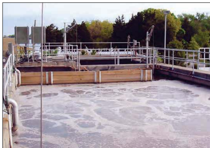
The aeration tank and anoxic zone baffles are an integral part of the MLE process.
