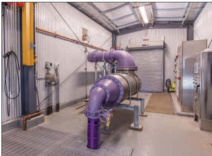
Reuse water supply piping to the golf course irrigation system, including a high strength ultraviolet disinfection vessel.
