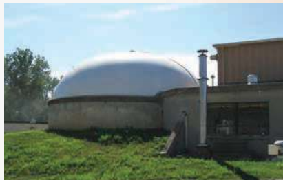
Digester Gas Holding Cover
