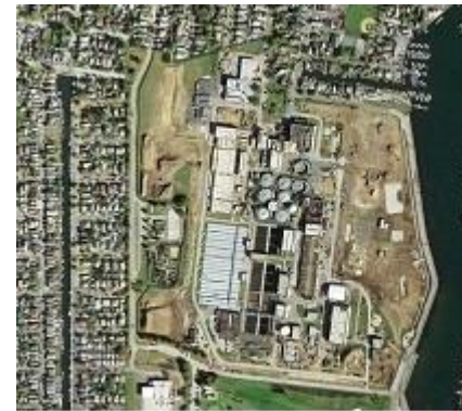
Bay Park WWTP
