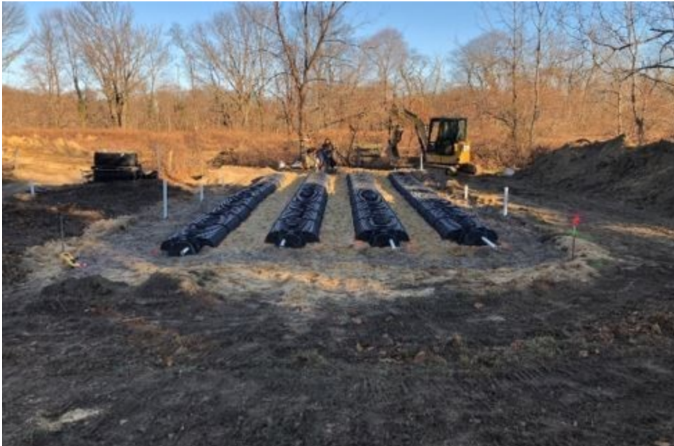
Installation of NRBs. Photo Credit: CCWT
