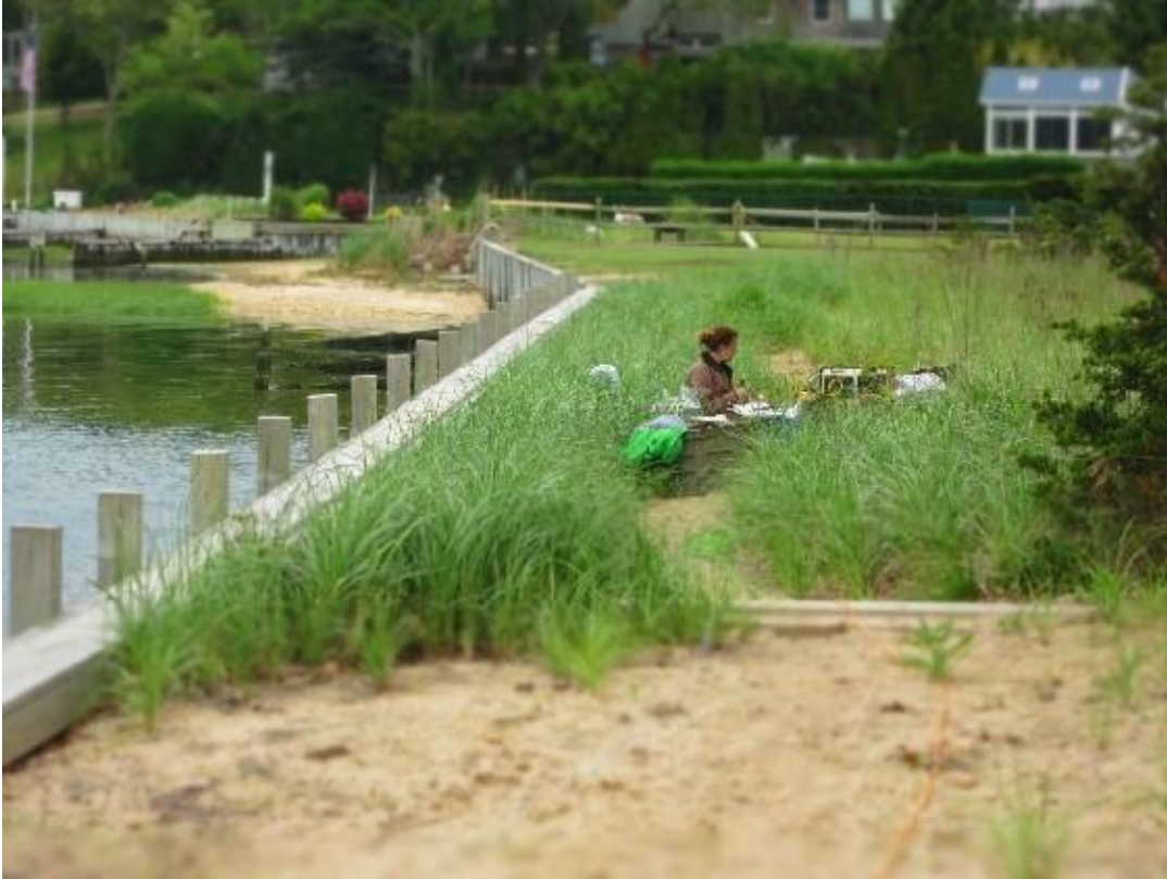
a bulkhead permeable reactive barrier test cell.
