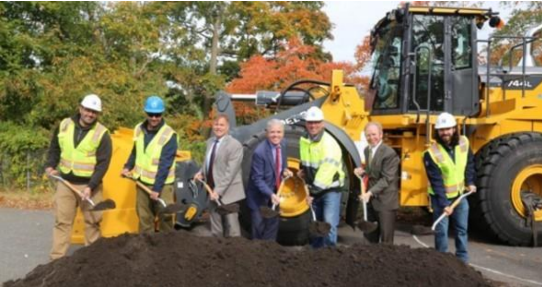
Sewer expansion groundbreaking in the Town of Babylon. Photo Credit: Suffolk County
