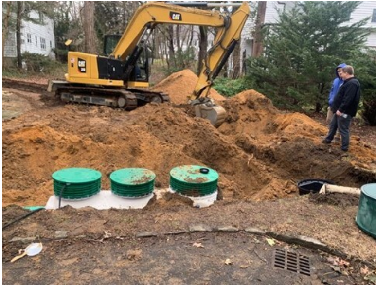
Installation of I/A OWTS at a residence in Manhasset. Photo credit: NCSWCD.
