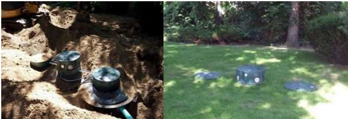
Innovative/Alternative Onsite Wastewater Treatment System Installation. Photo Credit: Suffolk County
