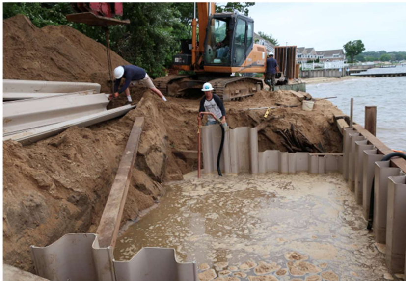
Installation of bulkhead PRB in Hampton Bay. Photo Credit: CCWT.
