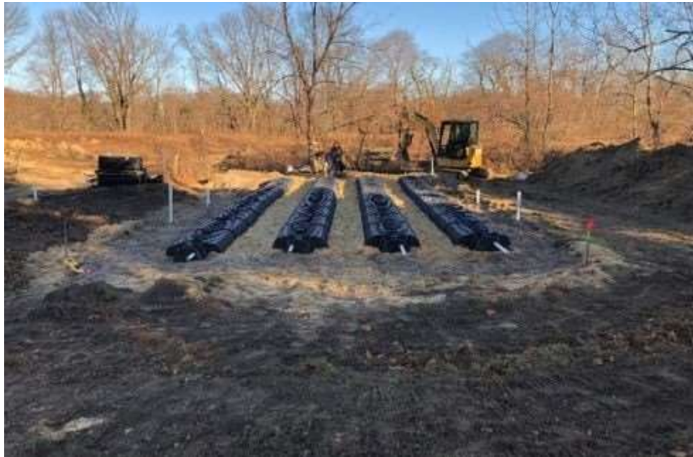
Installation of NRBs. Photo Credit: CCWT
