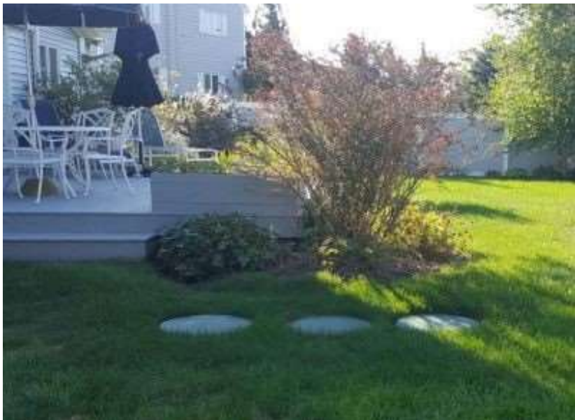
Innovative/Alternative Onsite Wastewater Treatment System Installation (Fuji Clean CEN Series) - Photo Credit: Suffolk County
