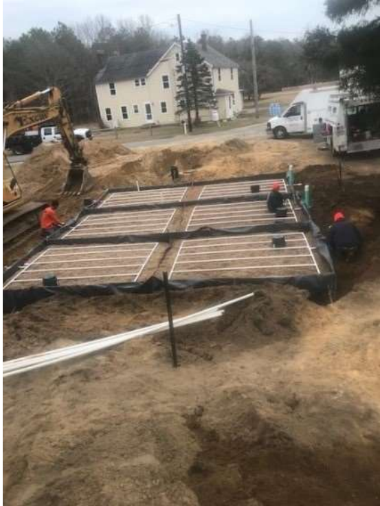
NRB test cells to determine optimum dosing rates. Photo Credit: CCWT
