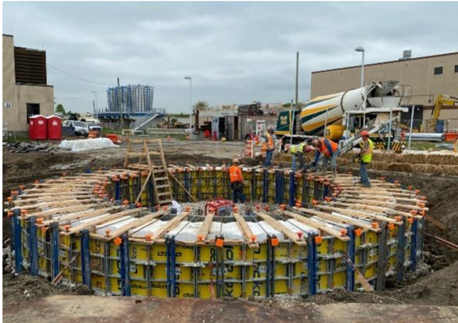
Construction on Bay Park Conveyance Project. Photo Credit: Nassau County
