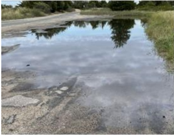
Louse Point Road Parking Area before and after. Impermeable asphalt was replaced with crushed quartz gravel to drain and filter stormwater. Photo Credit: Town of East Hampton
