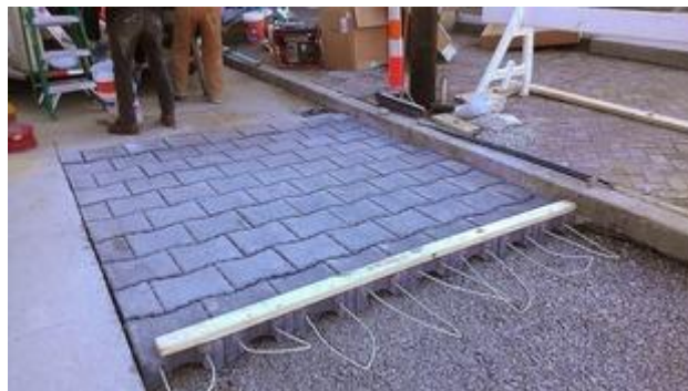
Permeable Pavement. Photo Credit: EPA
