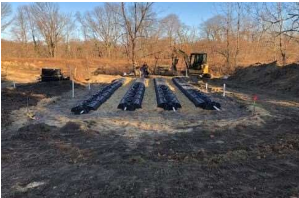
Installation of NRB. Photo Credit: CCWT
