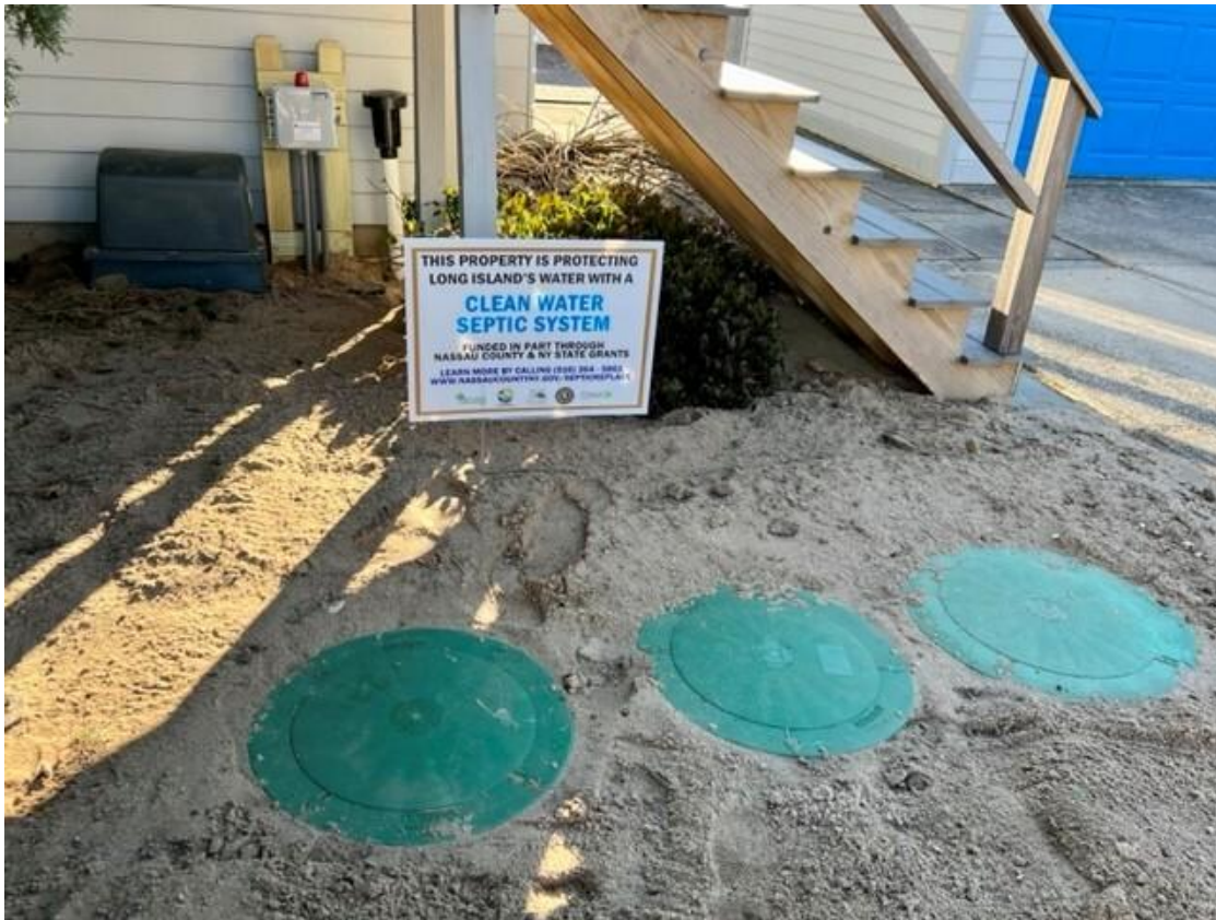
IA/OWTS System Installed. Photo Credit: Nassau County Soil and Water Conservation District.
